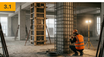
Reinforced Concrete Strengthening
