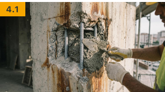
Concrete Damage Repair
